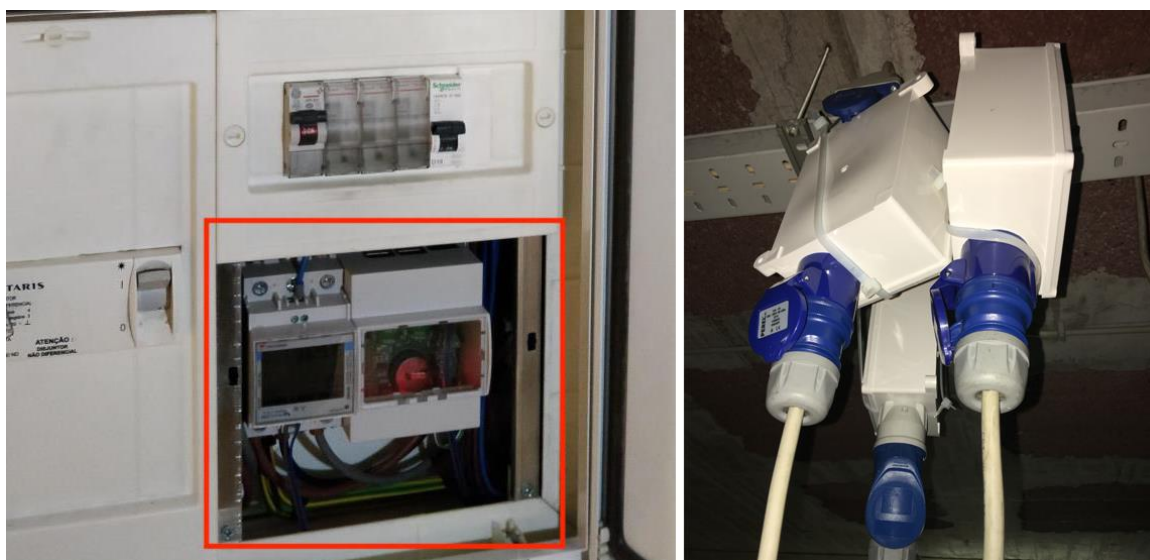
Figure 23. Energy Monitor and Gateway installation at TukxiTours (on the left) and Smart Plugs (on the right).
