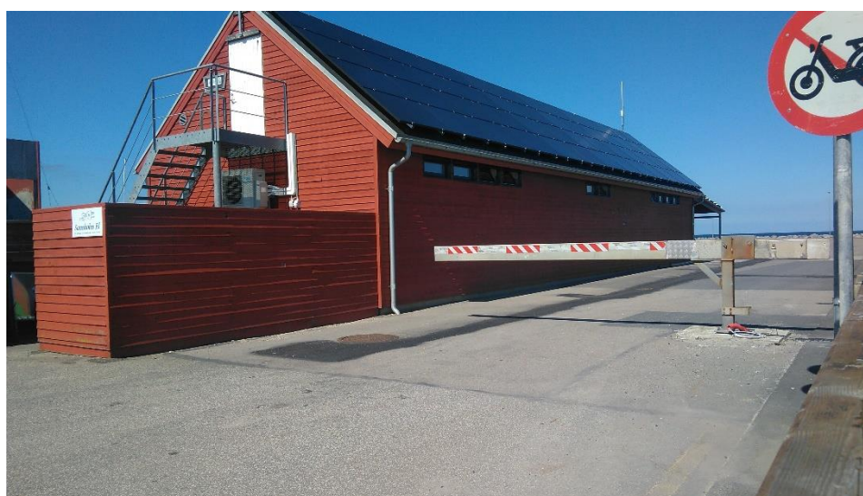
Figure 3. The service building. It contains showers, toilets, sauna, laundry, and a technology room. There are new PV panels on the roof and on a small roof at the end of the building in the background.
