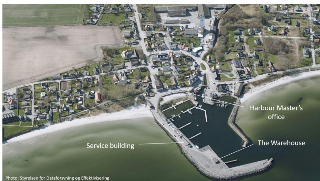
Figure 1. SMILE uses existing buildings on the Ballen marina. North is to the right, and the Southern Pier is the L-shaped concrete pier on the left side of the harbour.
