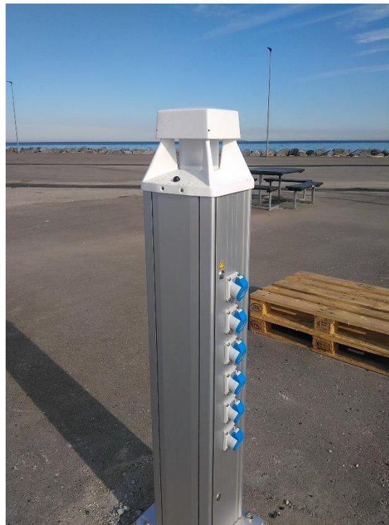
Figure 8. New socket stand. Each of the six blue sockets has a remote switch and an electricity meter. The tower contains a radio transmitter, which forms a wireless network together with the other towers.
