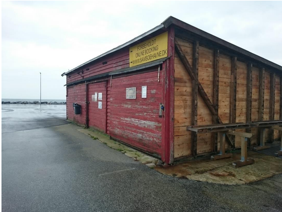
Figure 4. The Warehouse building before renovation.
